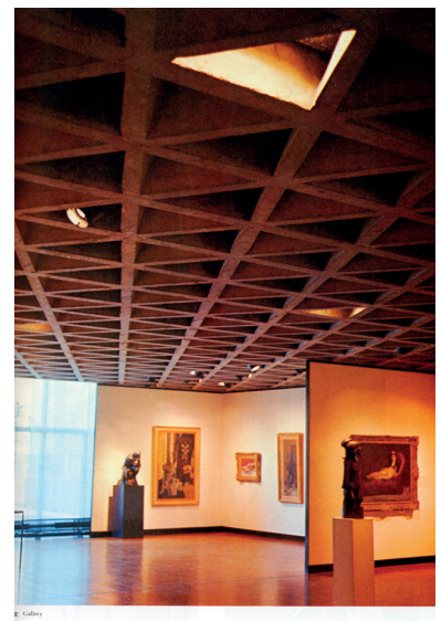
Kahn's inability to re-invent an 'Ordine' led him, in his Yale Art Gallery of 1951-3, to adopt the column-free spaces spanned by the 'space-frames' of August Komendant and Buckminster Fuller. These he 'monumentalised' (as they would never have) in wet-cast concrete.
