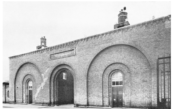
The 1814 Stables to the Royal Hospital at Chelsea manifest the wall as a unique succession of arched incisions worthy of an Egyptian 'door of appearances'. The entablature appears swallowed by the layers of wall in front of that the layer into which the doors are actually fixed.
